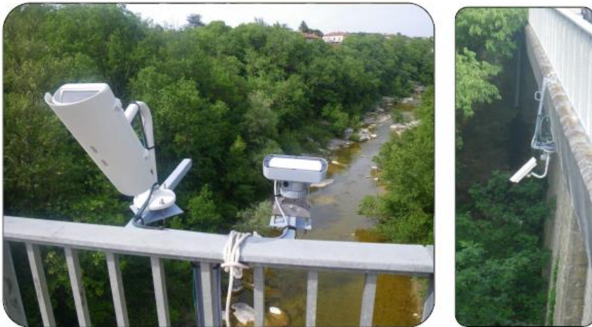
Camera and radar level gauge Auzon at Vogüé-Gare (INRAE)
